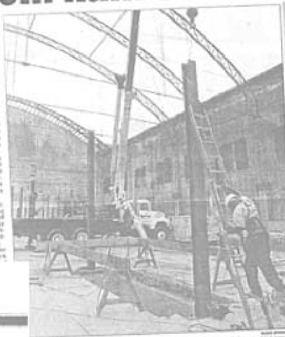
WORKING: Workers erect columns to support study of being built above parking area at the 130-year-old Clinton Armory near Myrtle Ave. in Fort Greene.
