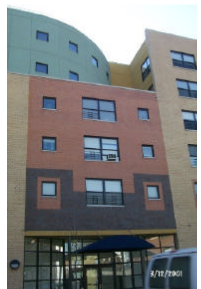
An 84-unit, low-income, rental property situated between Hoe and Vyse Streets in the Crotona Park section of the South Bronx, 950 Jennings Street has a $990,000 mortgage issued by CPC with 100% REMIC insurance.
